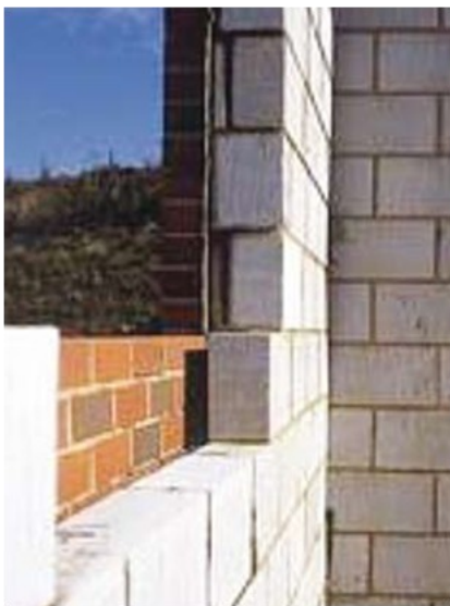
Modern cavity walls under construction
